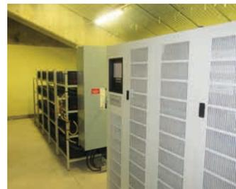
The stadium's lighting was not functioning because the battery bank (left) on one of the UPS units had failed unexpectedly. Eaton's team delivered and installed 140 replacement batteries and carried out a service test on all four UPS units (Source: Eaton)
