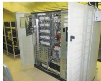
One of the four 400 kVA 9315 UPS units, which provide uninterruptible power in case one of the stadium's two generators fails (Source: Eaton)
